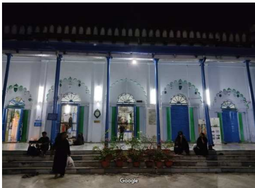
Rooms facing the courtyard
