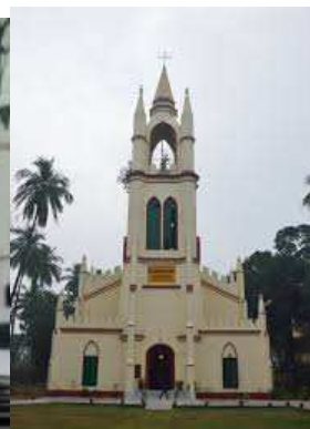
At the exterior of the church
